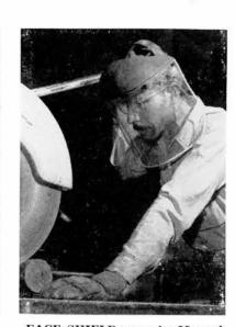
FACE SHIELD worn by Manuel G. Martinez, 2121, protects him from flying sparks and bits of sharp metal while sawing steel.
